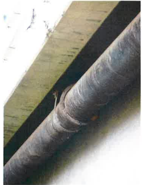
Figure 3 VVCSD 10" DIP SEWER LINE ON FLORADALE BRIDGE (1979-TODAY)
